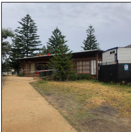
Figure 3: The informal works yard/facilities to the rear
