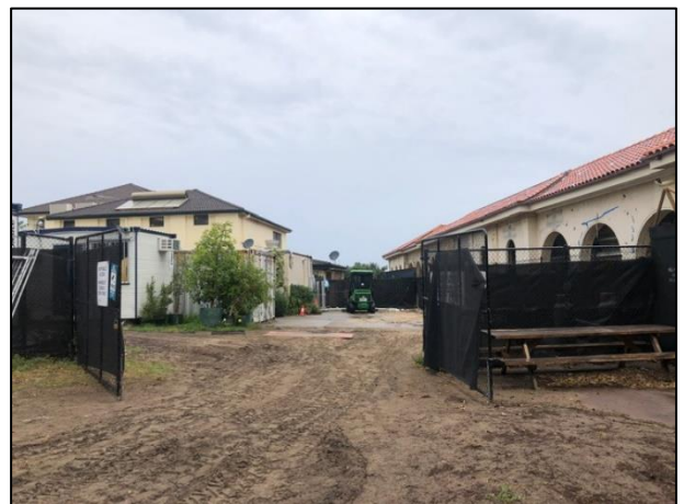
Figure 4: The existing building (left) as viewed from the rear, Bondi Pavilion is to the right
